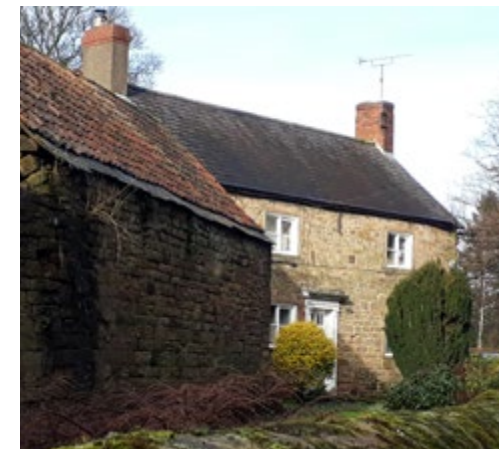
Traditional windows and doorcase, Stainsby
